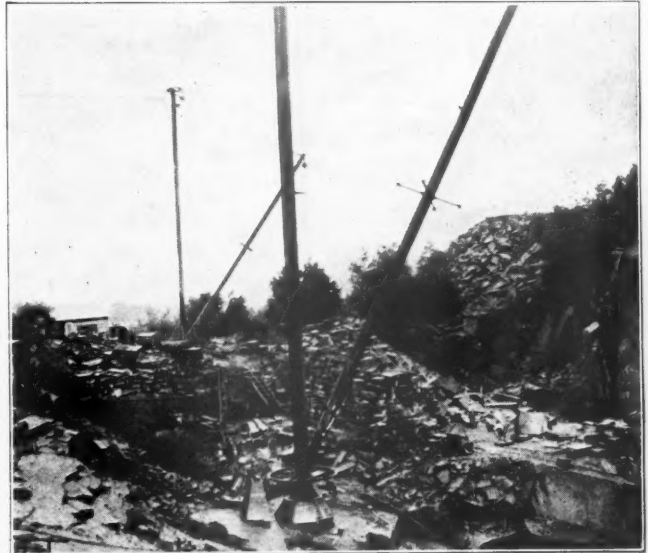
View of Two of the Derricks
